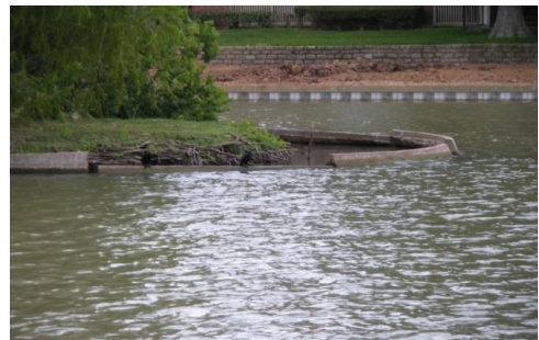
FIGURE 14: BULKHEAD FAILURE
