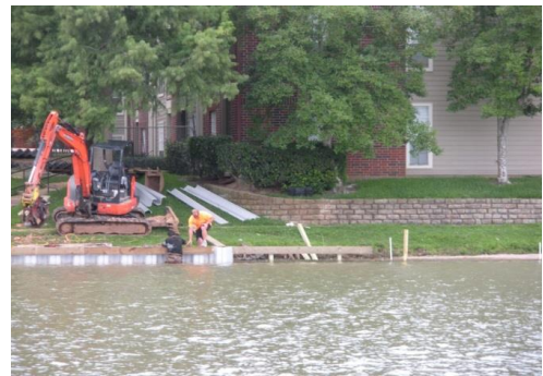
FIGURE 11: BULKHEAD REPAIR
