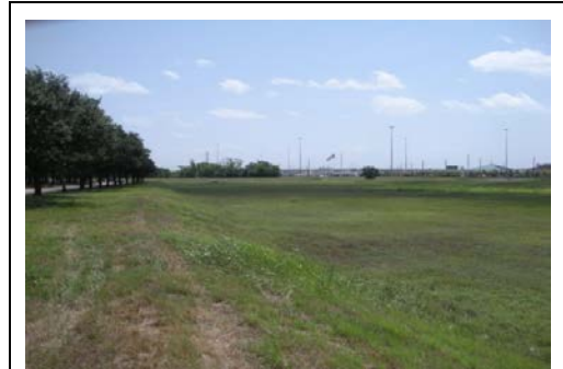
FIGURE 7: DRY DETENTION POND
