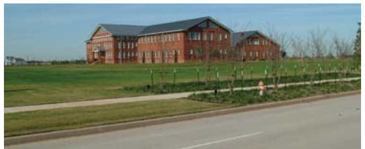
Future home of the Museum of Natural Science satellite, a three-way partnership between Sugar Land, the Museum, and Newland Communities.
