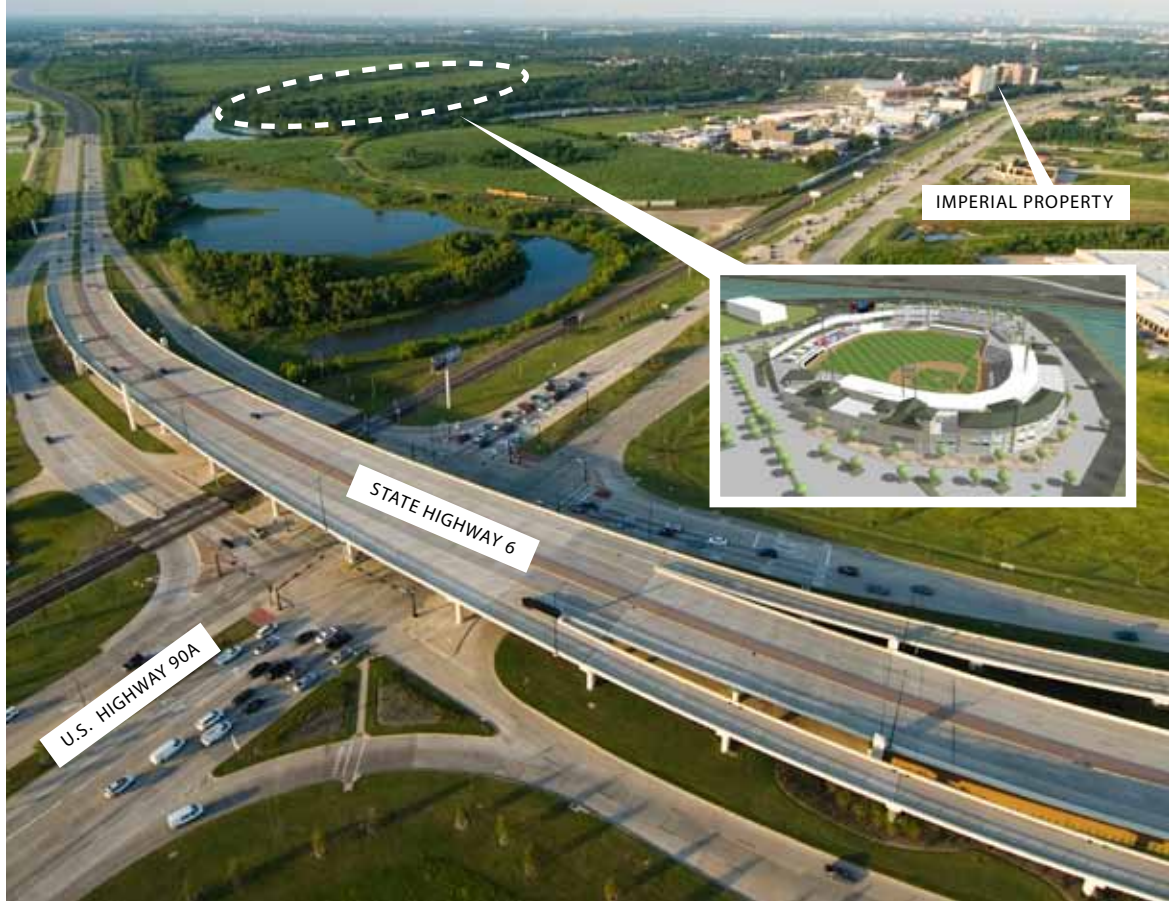
Sugar Land's professional minor league baseball stadium will be located northeast of State Highway 6 and U.S. Highway 90A, as approximated by the dotted oval. A proposed design is shown in the inset.
