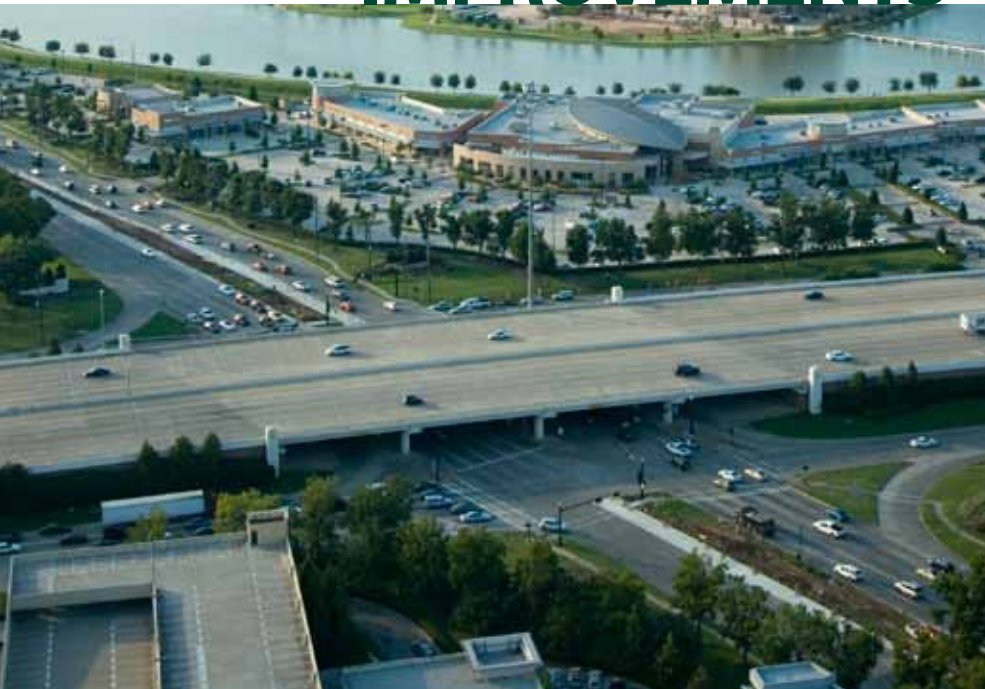
Looking north at US 59 crossing over SH 6.
