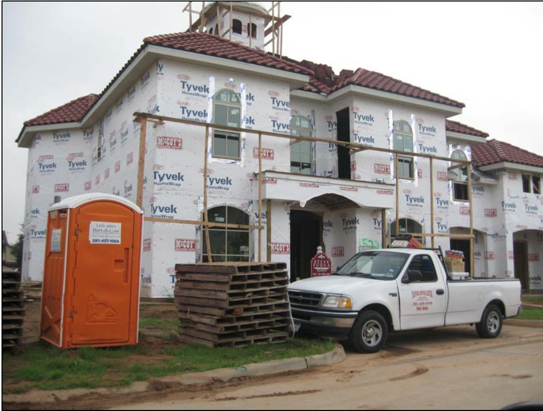
Home Under Construction
